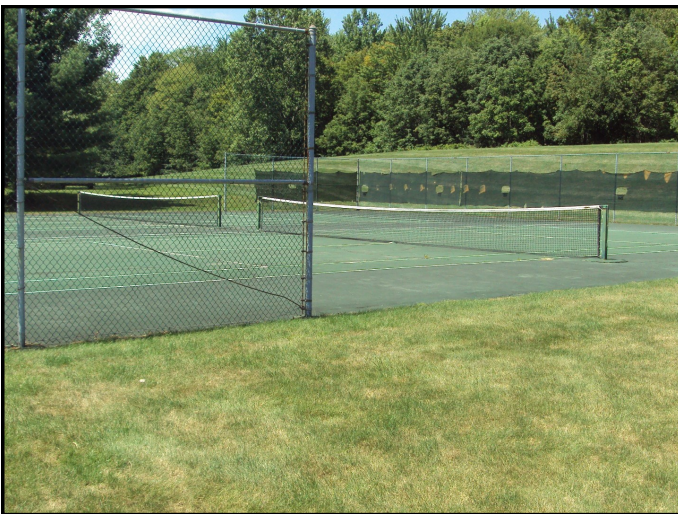
Tennis Courts—(Repairs recommended)
